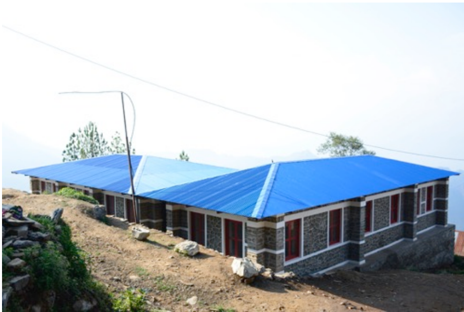
School opening in Bhorle/Rasuwa, on May 14th, 2016.
